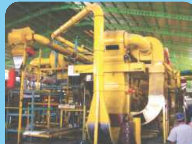
DUCTING PLAT BESI
